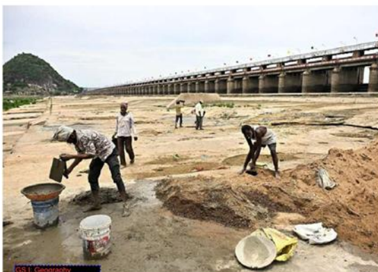
Labourers mix concrete and sand on the exposed Krishna riverbed in Vijayawada, for routine maintenance work during the seasonal low-flow period. The Prakasam Barrage is in the background. K.V.S.
